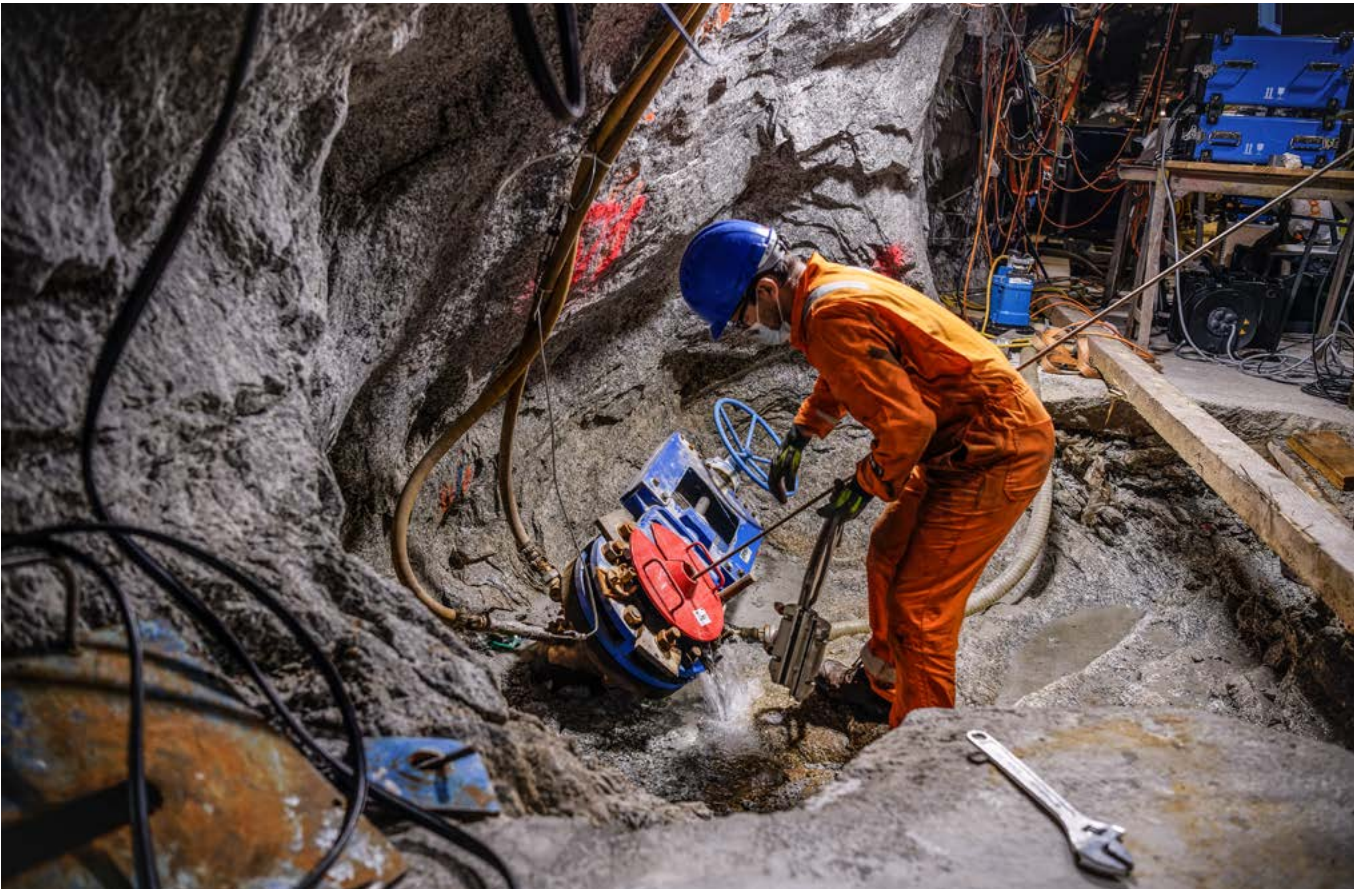
The most important part of the second underground lab will be the borehole (in the photograph with a red cover). Its diameter must be roughly twenty centimetres for the numerous sensors that record and monitor experiments to fit inside.
